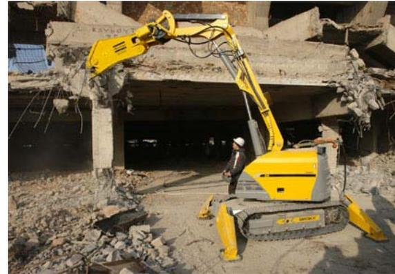
**Figure 4: Brokk 330 demolition robot [3].**
