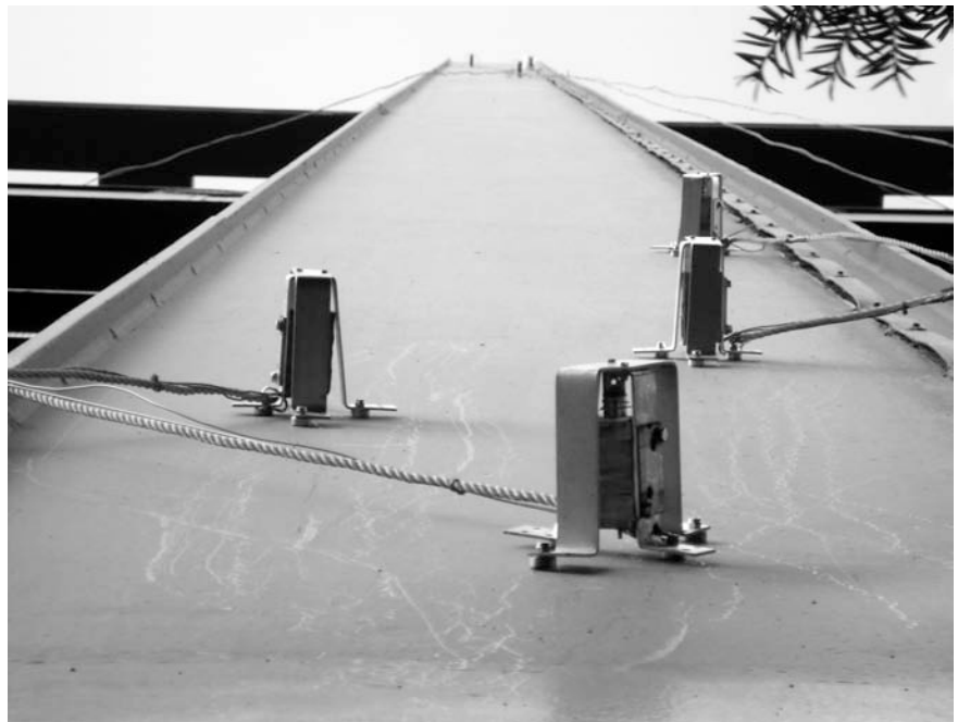
Fig. 2. Central pillar of the Fondation Avicenne building. Some "parasites" have already descended, while others are still located further up. (© Cécile Colle}{Ralf Nuhn.)
